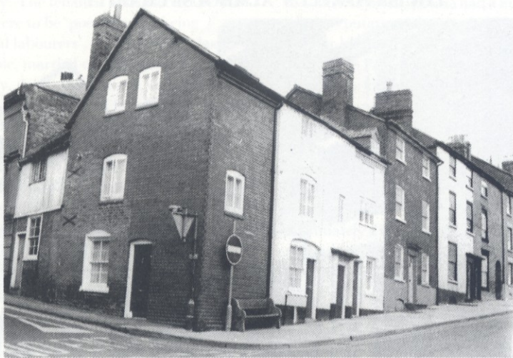
Restored houses on the corner of Brand Lane and Old Street
