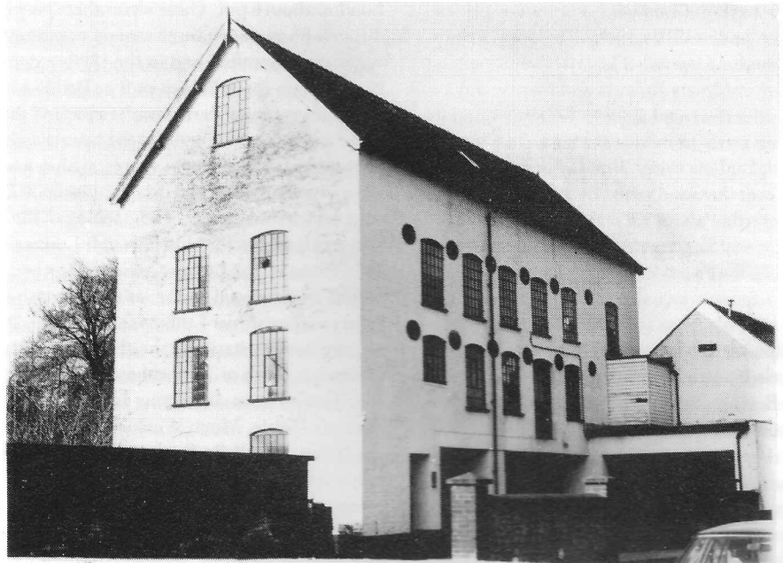
The Case Mill, Temeside, as it stands today
